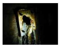
Figure 4. Seep Drains S-4 which is located in the southern Outlet Works Tunnel.
