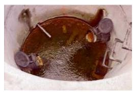
Figure 2. Manhole Drains The larger pipes with caps are the toe drains. Accumulated biofilm in the toe drains is visible.
