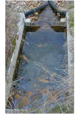
Figure 6. Manhole 14 weir (Right) Biofilm evident in weir and downstream.
