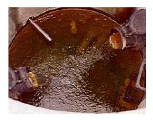
Figure 5. Manhole 14 (Above) Sump heavily populated by filamentous biofilm.
