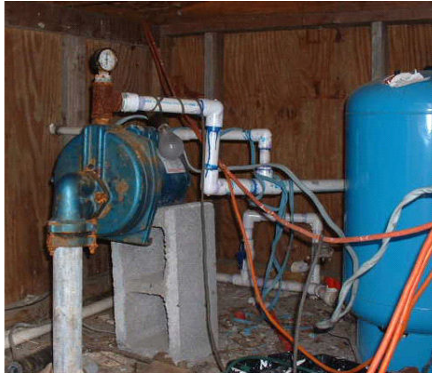
Figure 4.5. Two-inch well with in-line deep-well jet pump, Pender County
