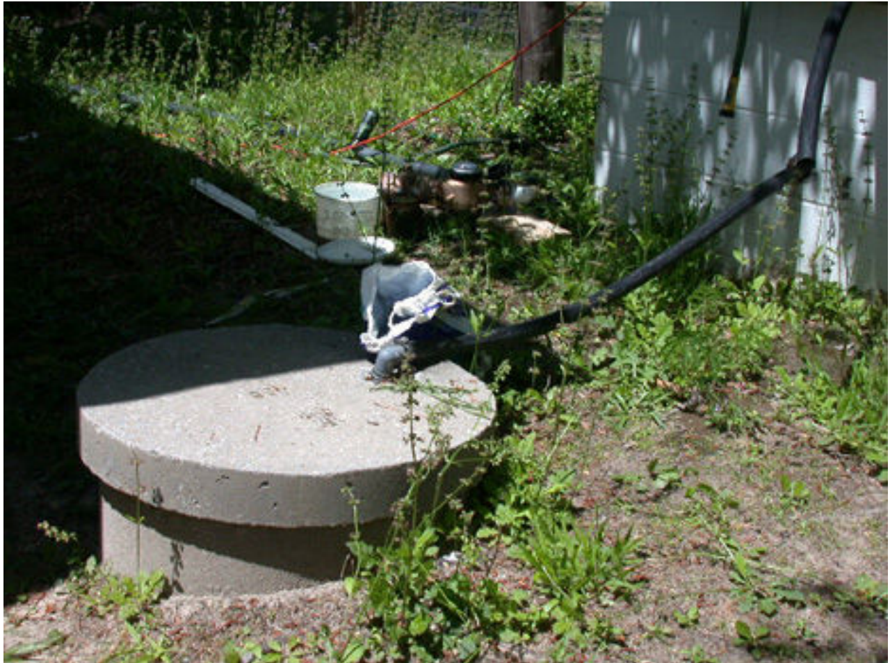
Figure 4.4. Bored well, Bogey Road, Edgecombe County
