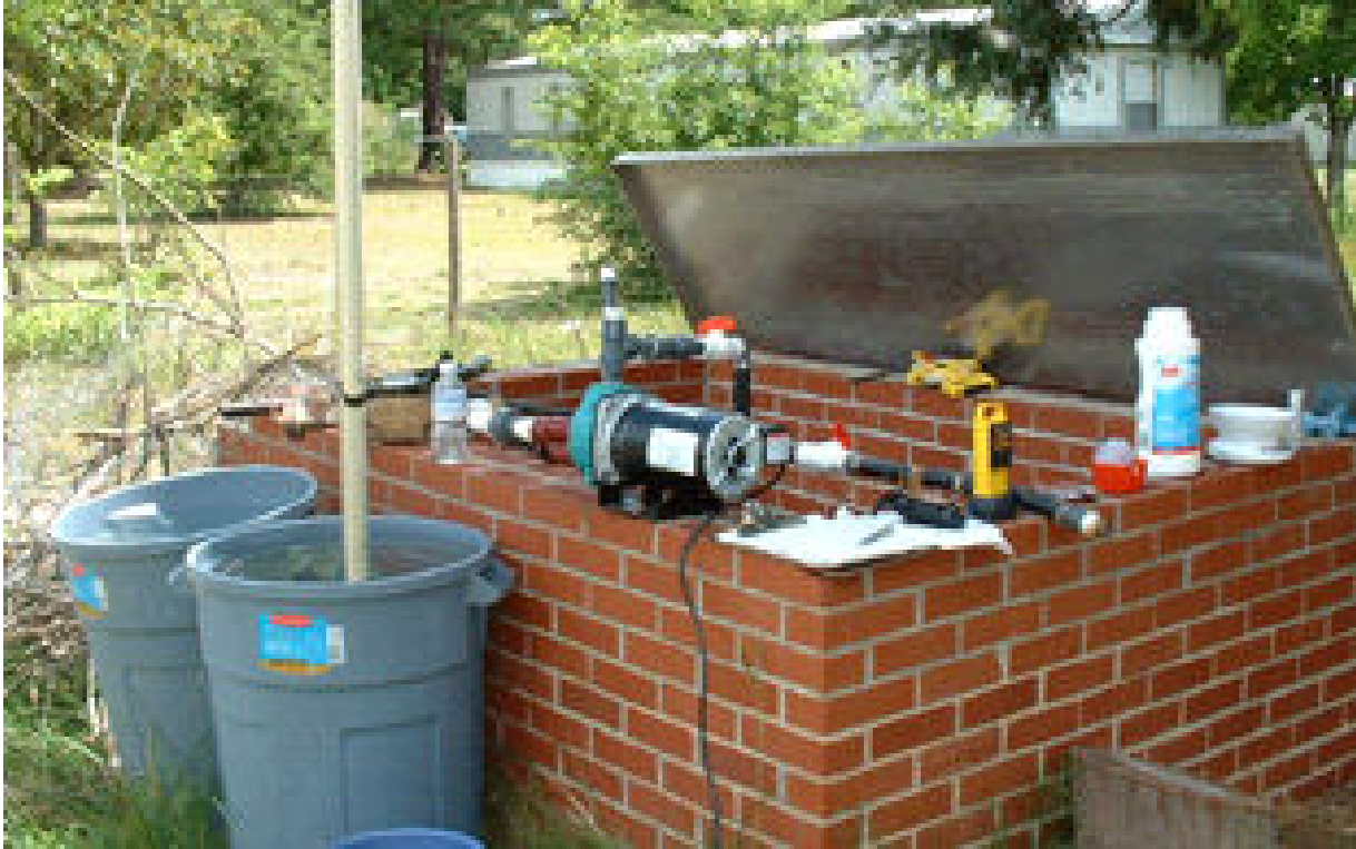
Figure 4.10. Bored well cleaning equipment at well Bogey A
